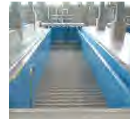
New Hardinge 600 filtration system
