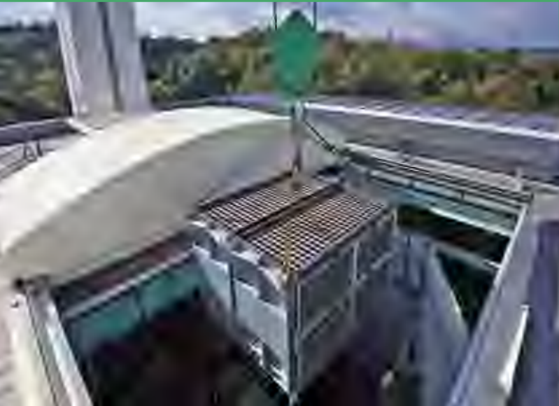
◀ Air preheater installation work (brought in from an opening in the building roof)
