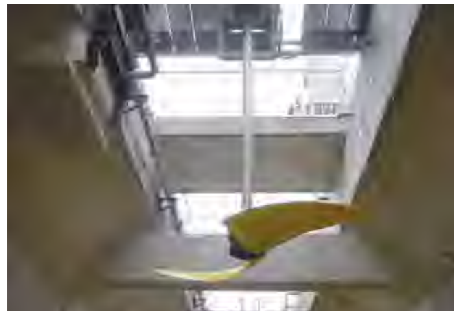
BB Mixer (Low power reactor stirring device) Has a simple structure, realizing energy saving with simple and easy maintenance
